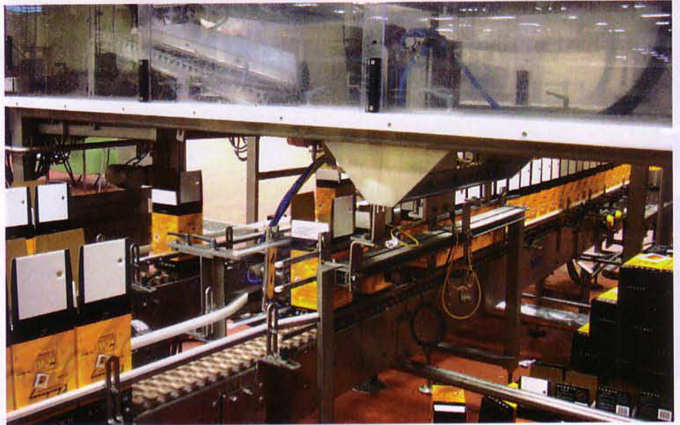
CLEAN FILLING. After being filled with a near-zero oxygen pickup, bags of wine drop down into cartons below.
